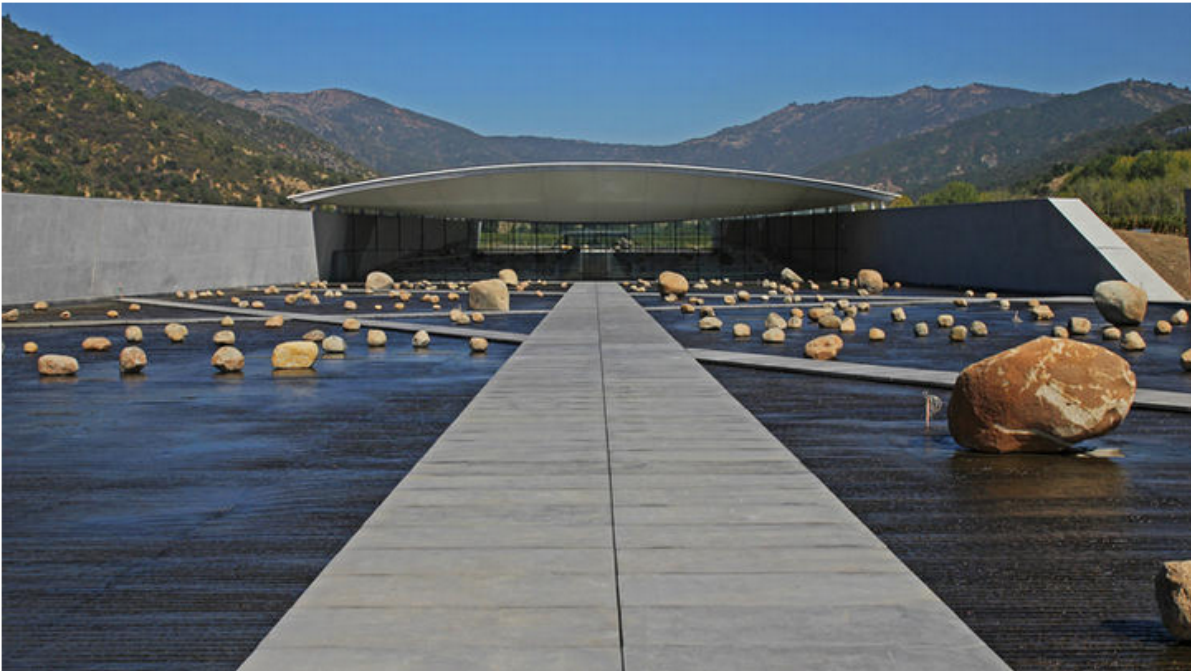
A dramatic water plaza punctuated by rocks greets visitors to Vik Vineyard in Chile's Central Valley. The winery complex was designed by Smiljan Radic, who did the Serpentine Pavilion in London in 2014. (Carolina A. Miranda / Los Angeles Times)
